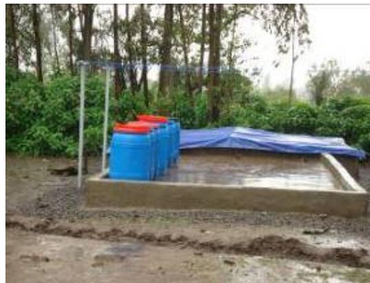
*A completed rinse area and covered evaporation tank.*
