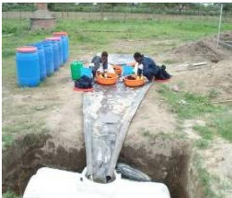
*Plastic sheeting and a 3,000 liter tank are used to handle DDT waste water in lieu of an evaporation tank.*
